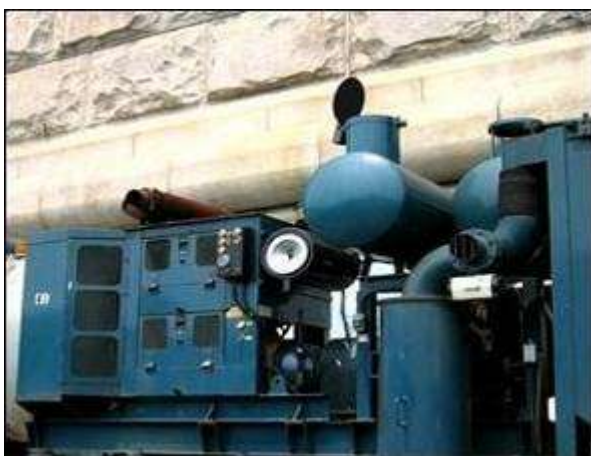
Figure 7.2.4.1.1: Muffler system
